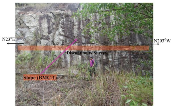
FIGURE 3. Discontinuity survey was conducted using the scanline method on slope BMC-1 underlying a 20 m diameter concrete water tank. The orientation of slope face is 293°/080°
