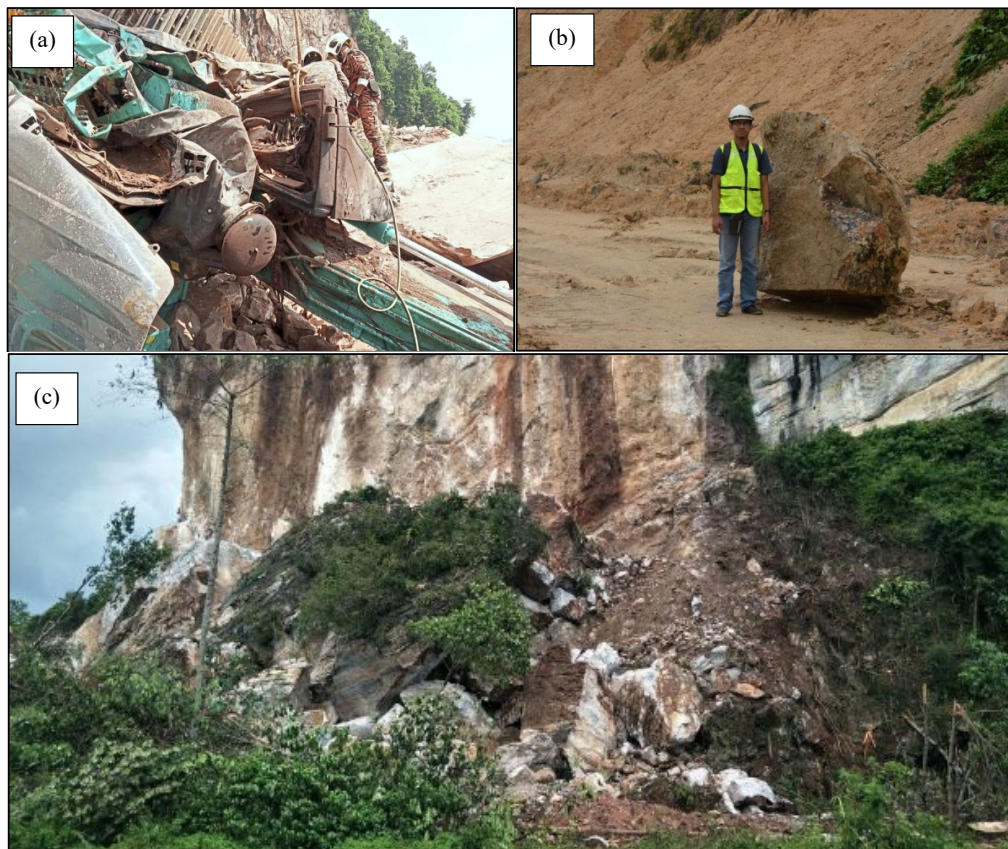
FIGURE 1. (a) shows a fatal rock fall incidence within a quarry in Kinta Valley (The Star Online, 2019), (b) shows a fallen granite rock within a construction site in Klang Valley in 2018 and (c) shows a large-scale limestone hill collapse forming multiple falling blocks at Kampung Kubang Rusa, Merapoh, Pahang (New Strait Times 2020)
